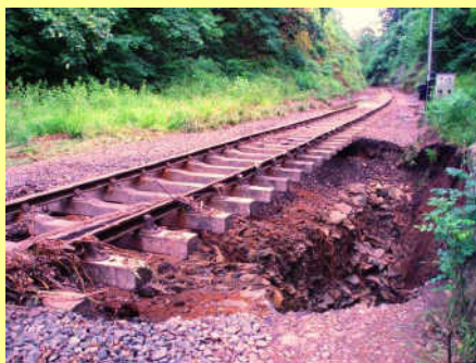
Damage at Eyemore cutting (left), repair work a few weeks later (middle) and also at Folly Point (right)
