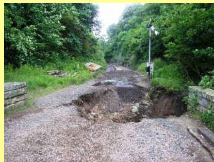
Damage at Eyemore cutting (left), repair work a few weeks later (middle) and also at Folly Point (right)
